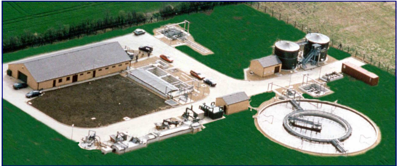
Ely Sewage Treatment Works
