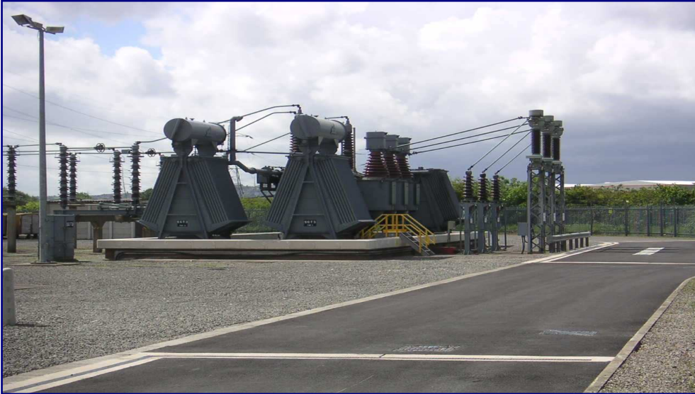
SGT3 Bund Wall Extension
