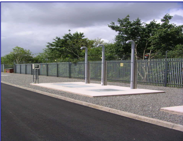
275KV - Retention Sperator
