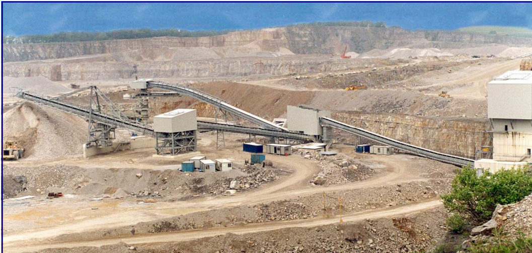
20M High R.C Crusher Structure
